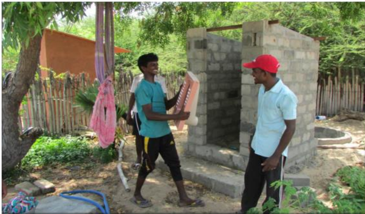
Building latrines in Sri Lanka.
